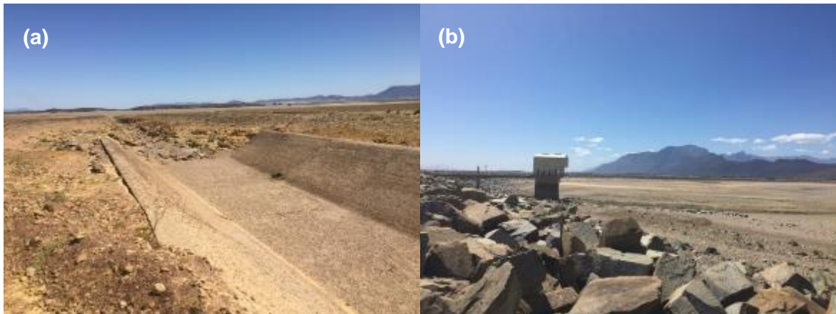
Figure 3: Canal feeding Voëlvlei Dam (a) and a dry Intake tower at Voëlvlei Dam (during the summer of 2016 (b))
