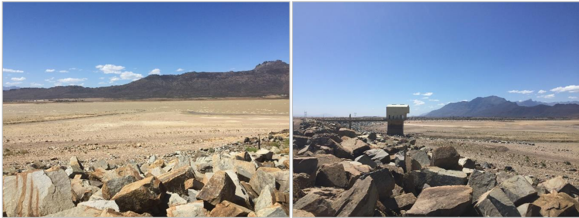
Figure 27: Images of the low water levels of the Voëlvlei Dam
